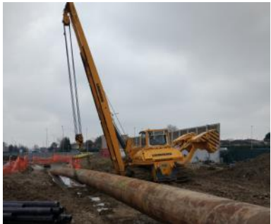
Pullback DN850(34") pipe string
