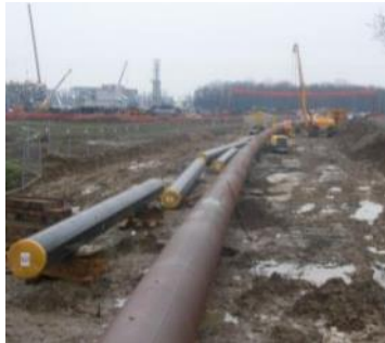
Pullback DN850(34") pipe string
